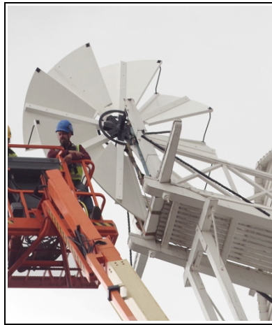
Fantail arrives ready for hoisting into position
