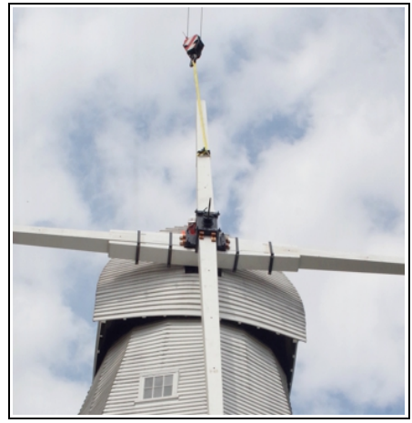
Stocks fixed into canisters
