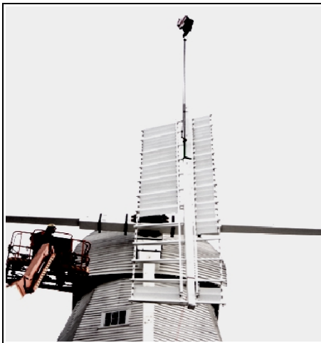
Sweep being hoisted
