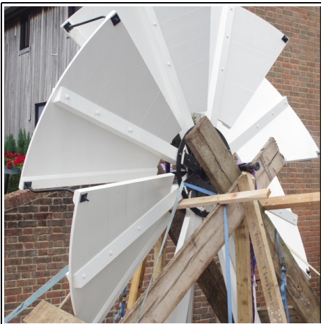
Fantail arrives ready for hoisting into position
