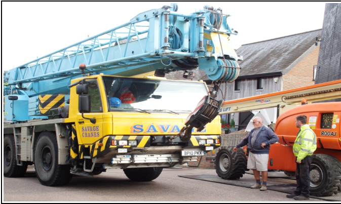
Tight fit for the crane and cherry-picker
